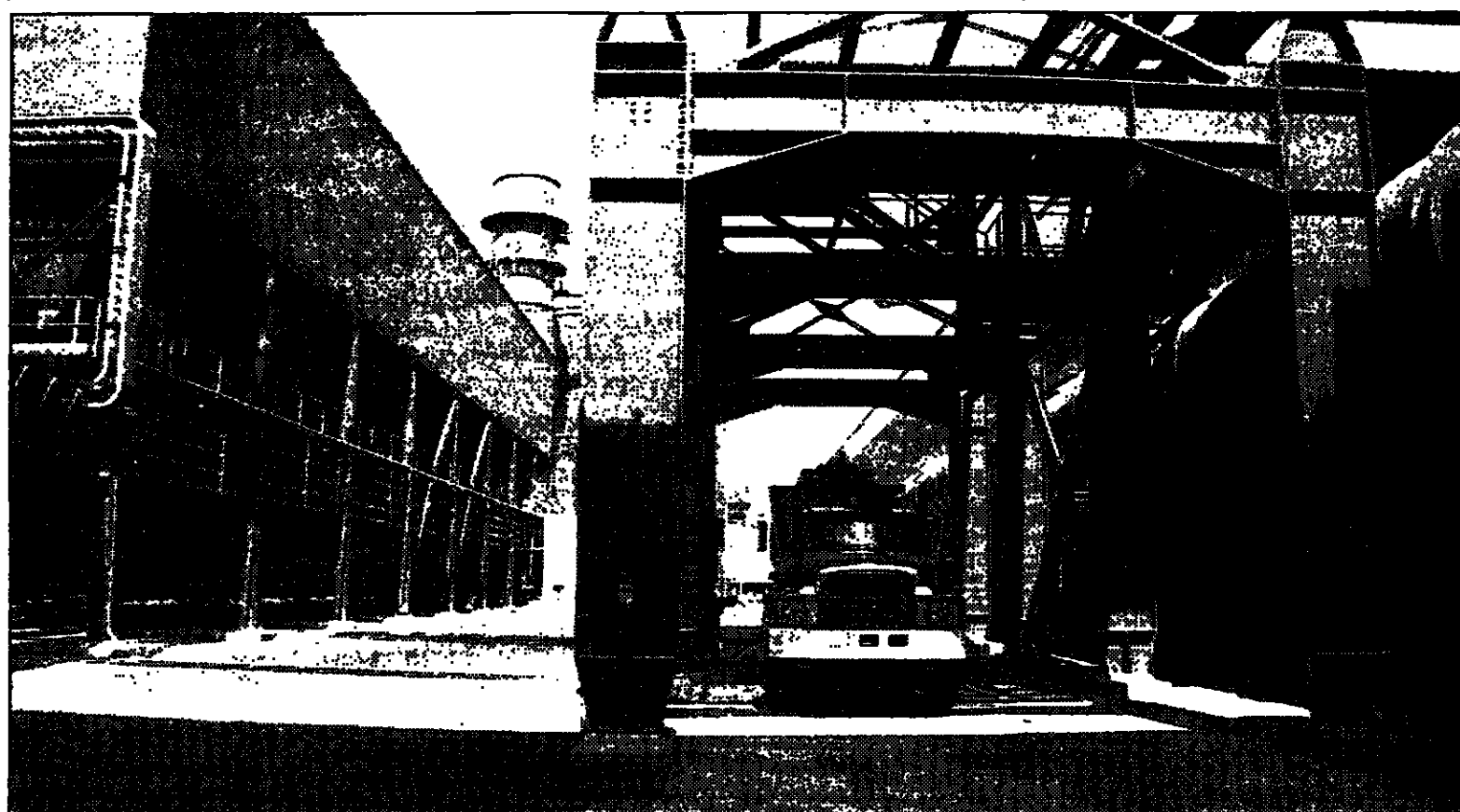
Gas-cleaning plant and solid-bath unloading station for the new No. 4 potline.
